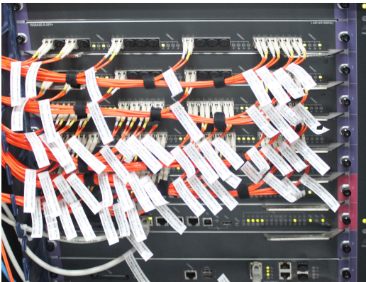
Figure 12-5 Optical fiber management
