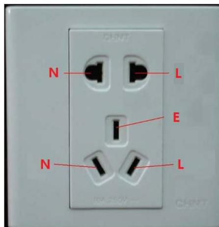
There is a shortcut way to check whether the connection of these cables is standard or not (not the accurate check).
