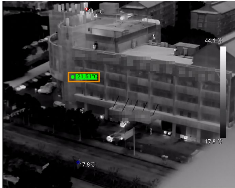
Figure 4-6 Real-time spot temperature measurement
